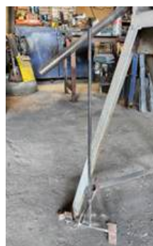
Fig. 6. Construction of the paddle agitator in a blacksmith workshop - Own elaboration
