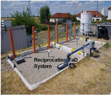
UFZ Ecotechnology Research Facility, Leipzig, Germany
